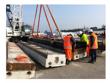
Each test sample is made up of two 10m long concrete beams jointed together as they are lowered into the shaft. Once installed, the jointed beam is secured in place using multiple hydraulic rams.
