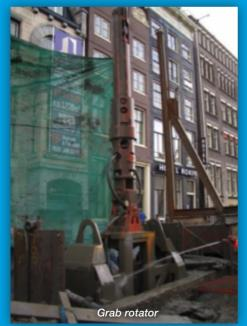
The **Grab Rotator**, a more recent development, has allowed accurate wall excavation by grab to 60 m - 80 m. In finer soils - where excavation by grab has significant advantage to the mill - **using a grab brings very substantial cost savings.**
